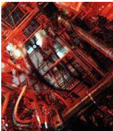
A fractionation column is charged with pyrolyzed plastic waste in order to precipitate various volatile components. (Photo: Peter Allert)
